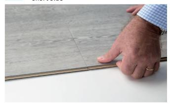
Continue pressing until the two planks are flush along the end joints.
