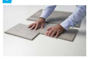
6 Continue sliding until the planks are fully separated
