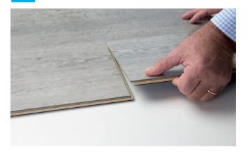
4 Press with your thumb on both ends of the short side
