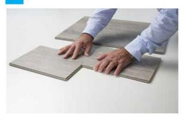
6 Continue sliding until the planks are fully separated
