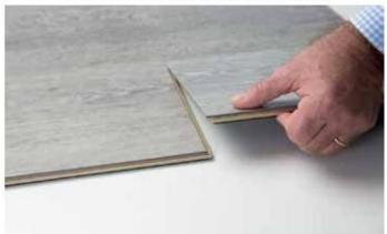
Press with your thumb on both ends of the short side
